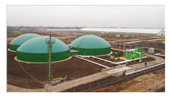
Figure 8: Enclosed Bio Gas Tanks
