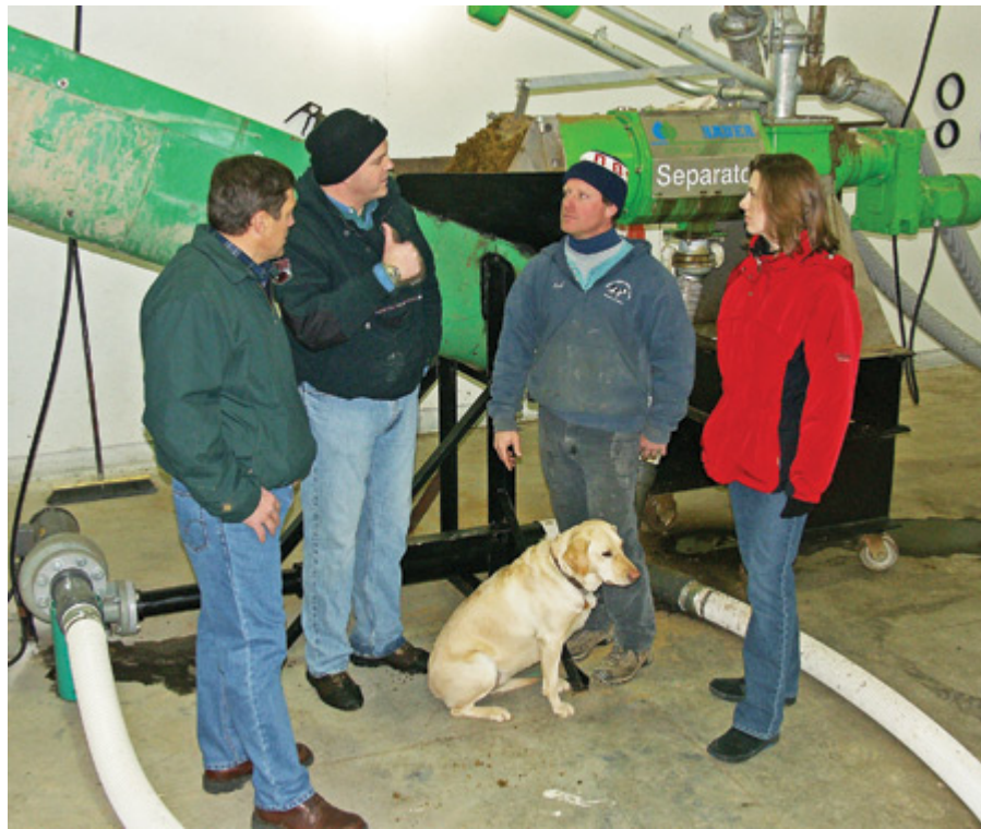
1. Tanks for the manure. Steve Dvorak (far left), who designed the digester at Blue Spruce Farm, Dave Dunn, Earl Audet (with Sierra at his feet), and Melissa Dvorak discuss the separation process, which divides liquids from solids after the manure spends 21 days in the digester. Courtesy: CVPS
